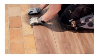
To fit the last row of panels you will usually need to cut them in. Do this as follows: lay a panel on top of the previous row with the groove towards the wall, lay another panel upside down up to the edge of the wall and mark the panel underneath. Cut the panel to size and fit the last row.
