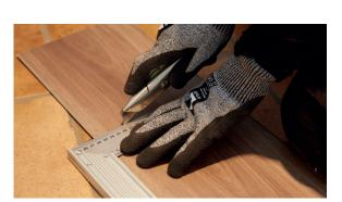
In places where it is too difficult to install the EVF Moduleo® LayRed® panels with the tapping block (e.g. against the wall), you can tap them together using the pull-bar and a hammer.
